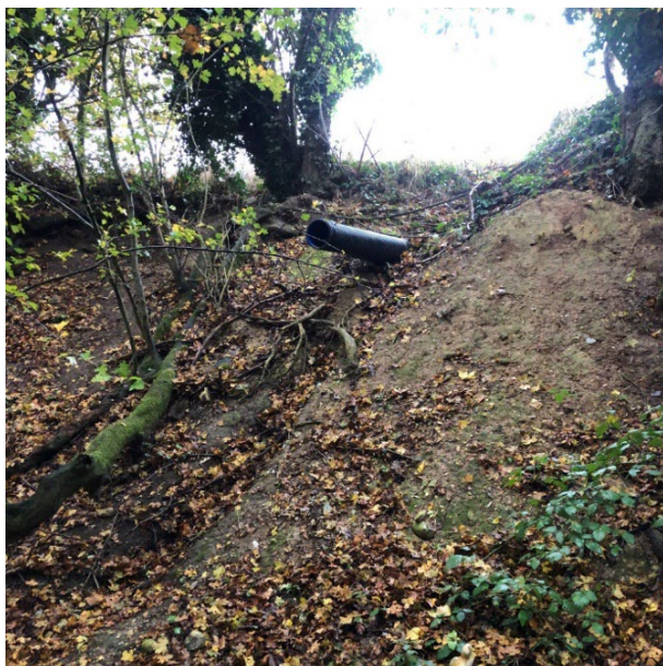
Photo 1 - 150mm Drainage Pipe discharging into hollow
